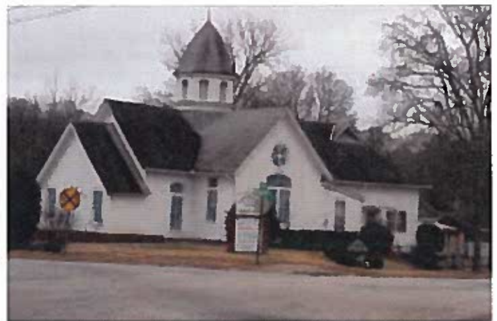
John King built Unity Methodist Church in 1903. Today, the building serves as a Baptist church for a Hispanic congregation. Photo by Jeanne Cyriaque
